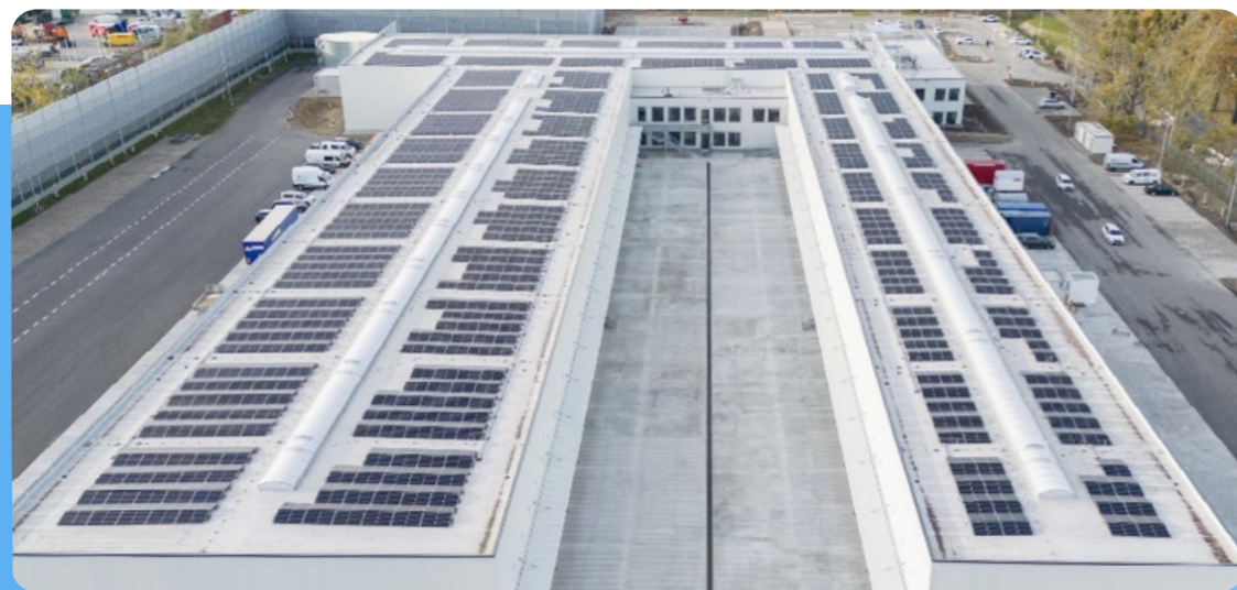
GLS Hub with solar panels in Potsdam (close to Berlin, Germany)
